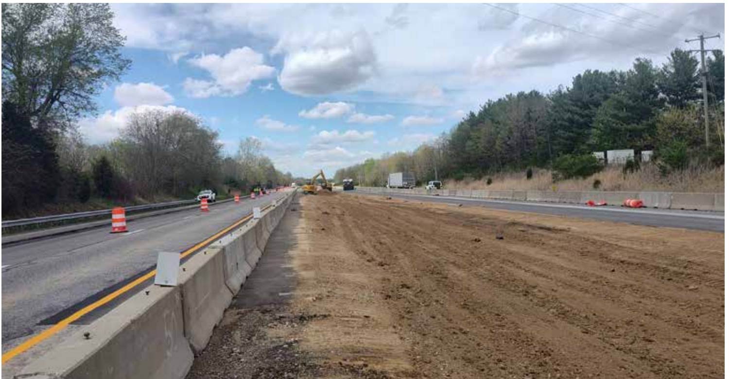
John R. Jurgensen Company working on I-74 in Greensburg, IN
