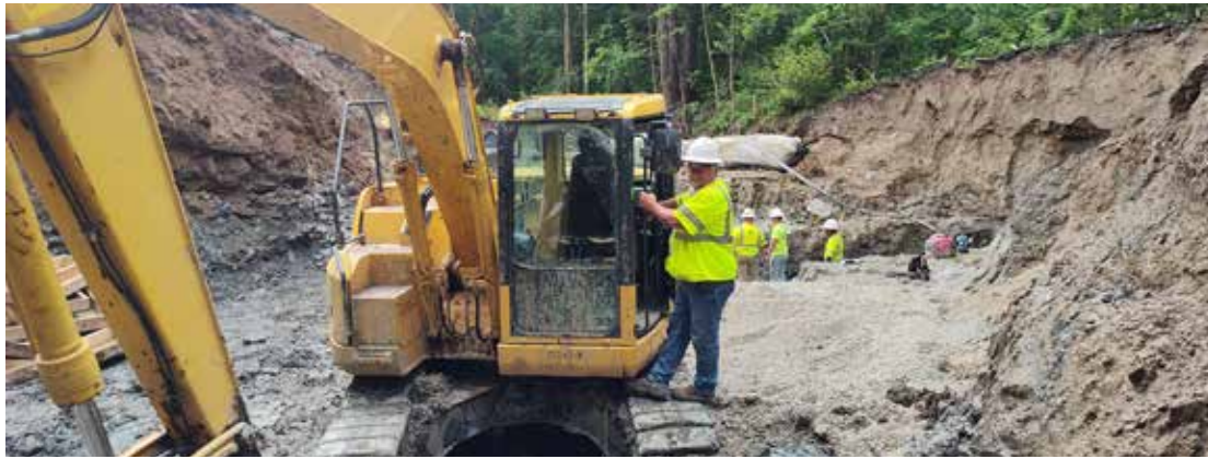
Jerry Wells, Morphe Construction in Mt. Carmel, IN
