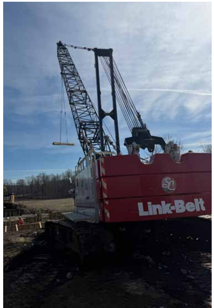
Jim Smith Contracting bridge work in Fredonia, KY
