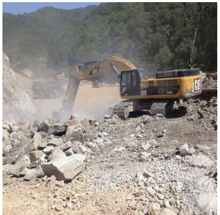
Hi-View working on the Mt. Parkway project in Morgan County, Kentucky.
