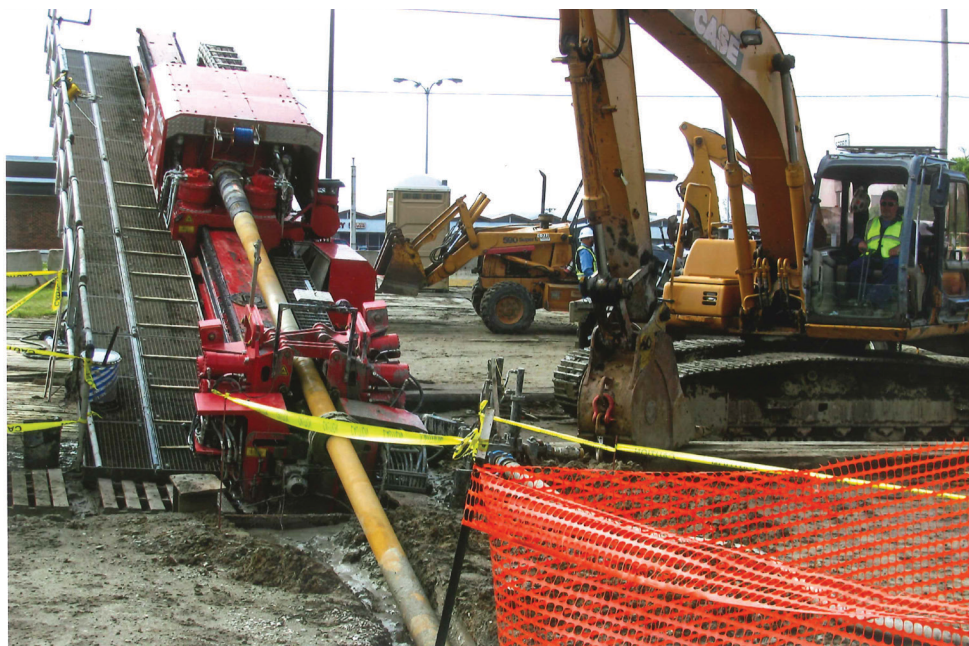
InterCon Construction boring under the Ohio River in Owensboro, Kentucky
