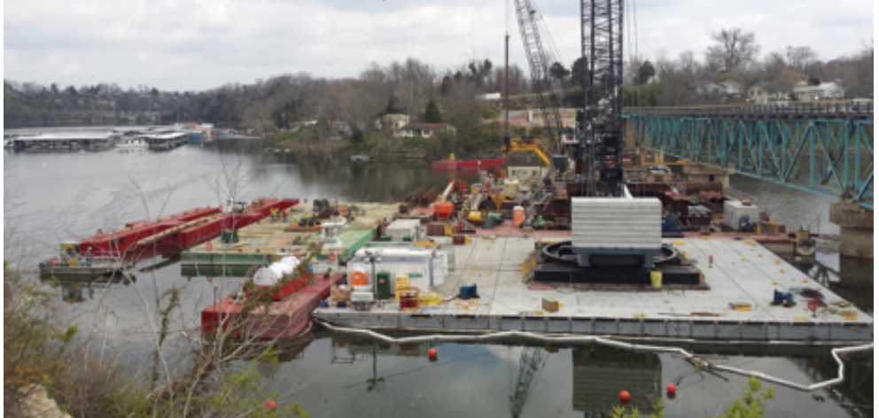
Walsh on Herrington Lake project in Mercer/Garrard Counties, Kentucky
