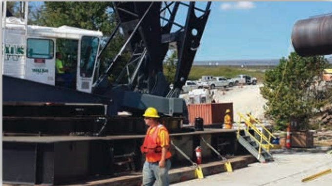
Walsh on the Garrard/Mercer County line bridge project over Lake Herrington.
